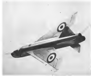
ENGLISH ELECTRIC P.1A has rounded leading edge of wing incorporating curved canards for enhanced lift. In this photo, demonstrator pilot R. F. Bennett was working turns low over the field at Farnborough pulling 6 Gs.
